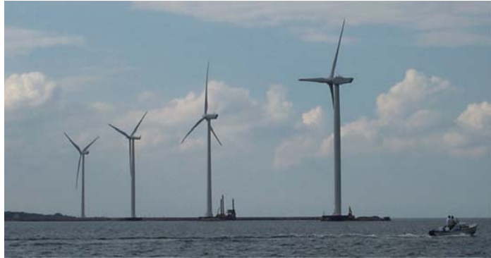
Figure 1: A cluster of four >2 MW semi-offshore turbines in Frederikshavn, Denmark.
